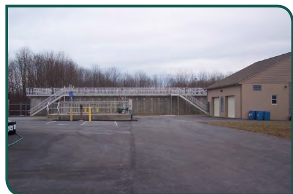
Fairfield Municipal Authority Sewer Treatment Plant
