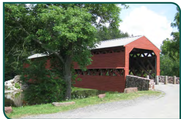
Sach's Covered Bridge, Freedom Township
