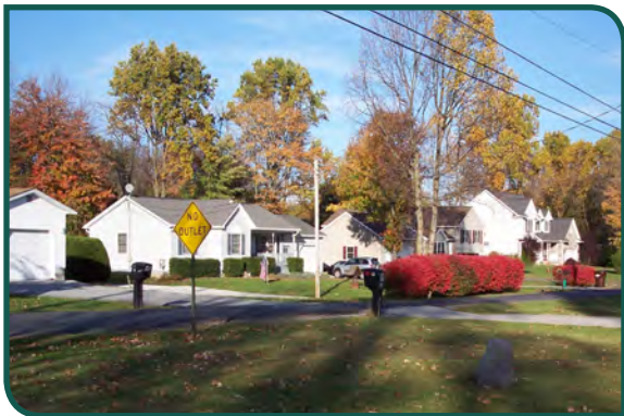
Existing residential neighborhood, Carroll Valley Borough
