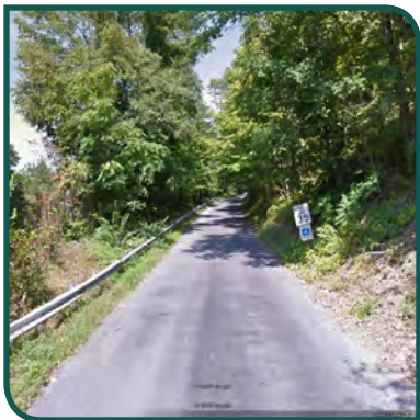
Steep slope setting along Steelman Marker Road, Liberty Township
