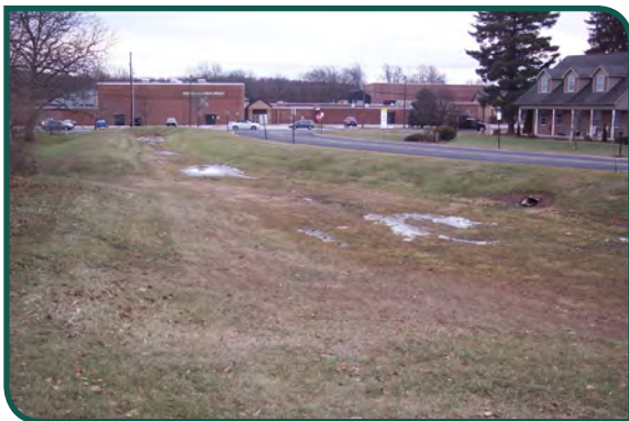
Stormwater management basin, Beechwood Development, Hamiltonban Township
